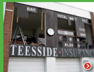
Removal of existing fascia and framework
